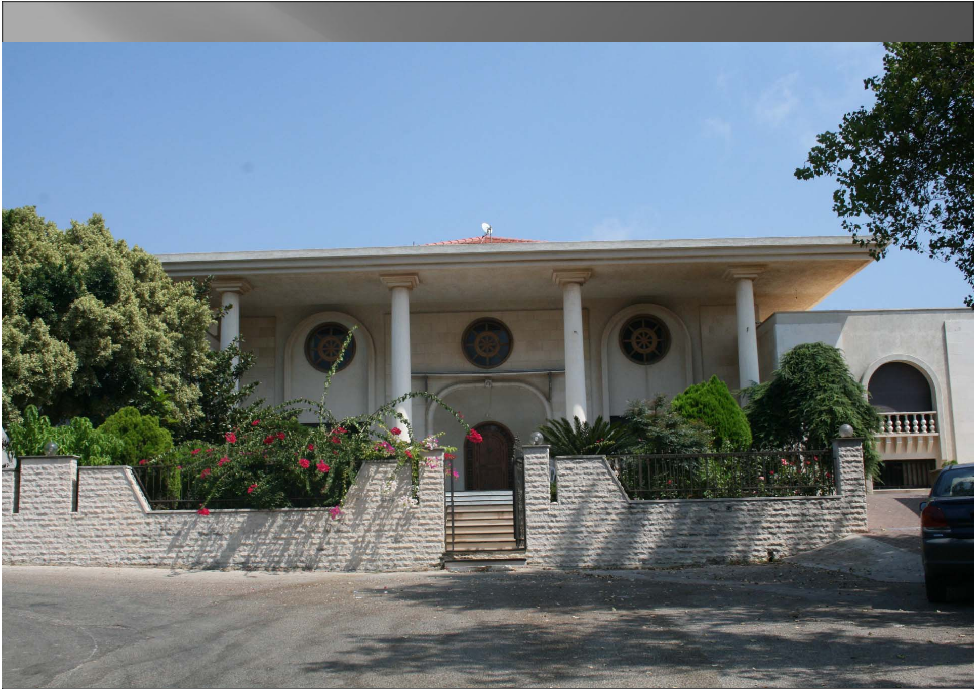
Hoda's home in Hamat. Her original home on this site was burned down in a skirmish. Sabah Abi-Hanna designed this home for her.
