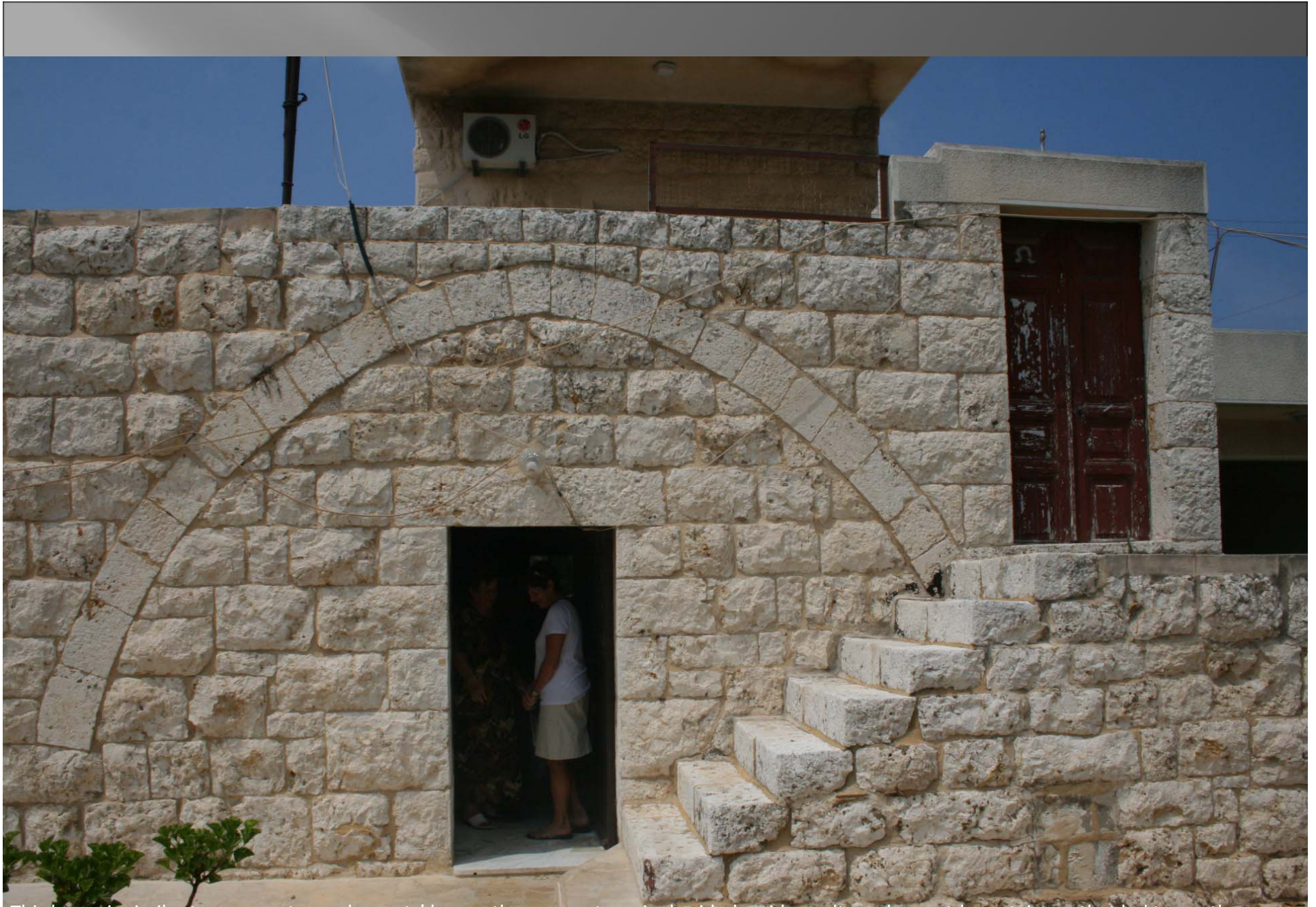
This home is similar to our great-grandparents' home: there were two single side-by-side vaults and an outdoor stairway that led to another room. As I understand it, the upper room of our great-grandparents' home was right on top of the roof of the other structure but there was not another doorway and structure to the upper side as shown in this home.
